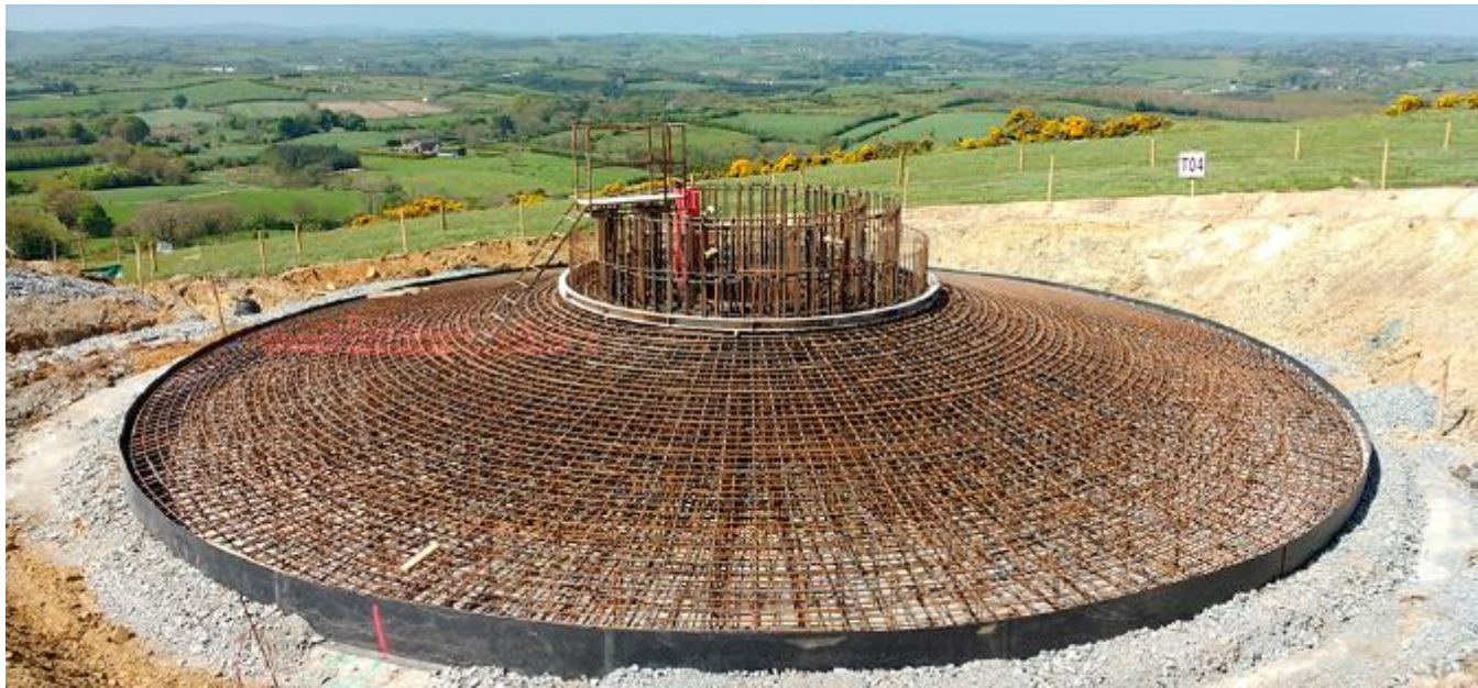
Figure 2.2 Sample Image of Turbine Foundation Anchor Cage
