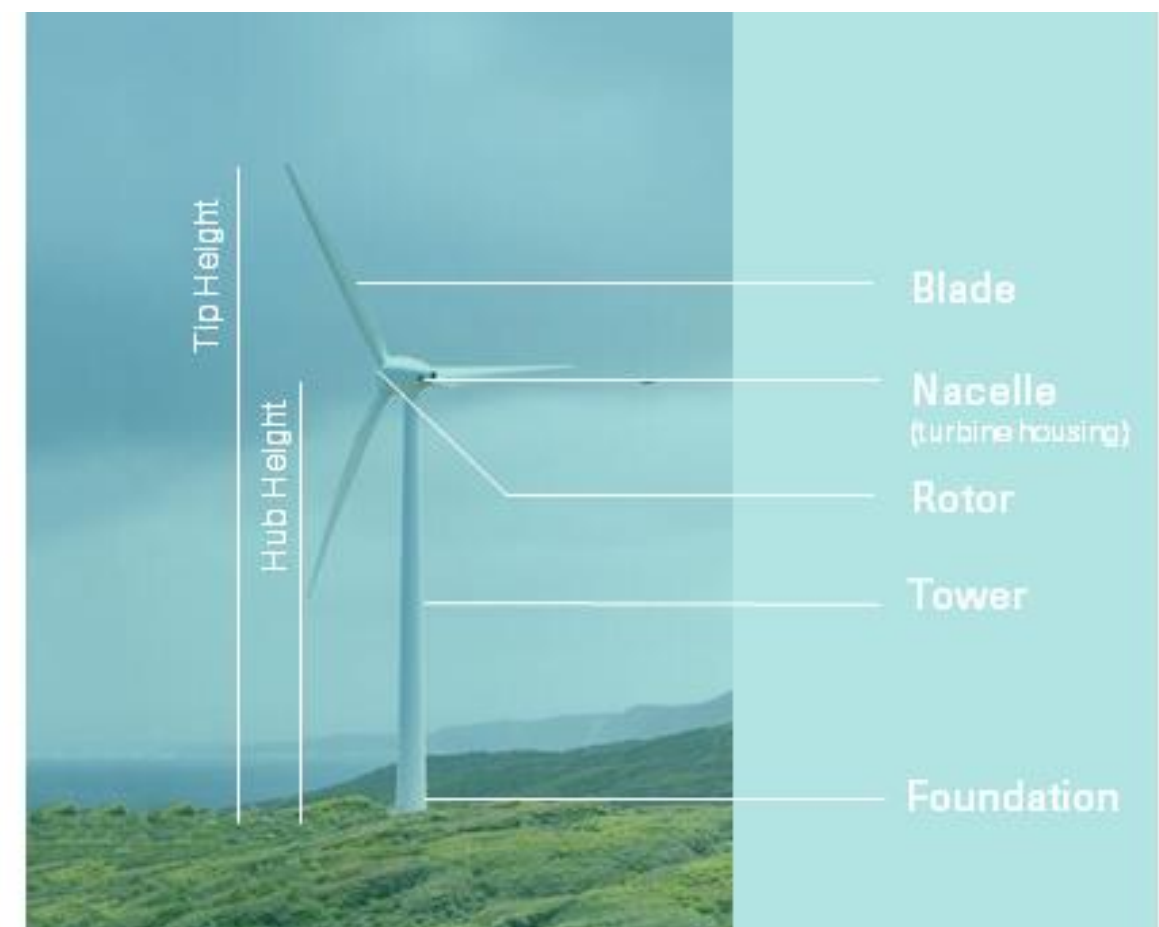
Figure 2.1 Turbine Components
