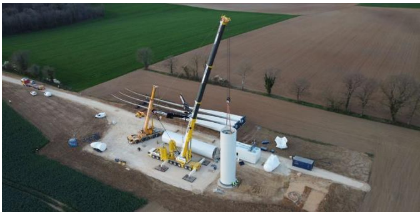
Figure 2.3 Sample Image of Turbine Hard Standing Area
