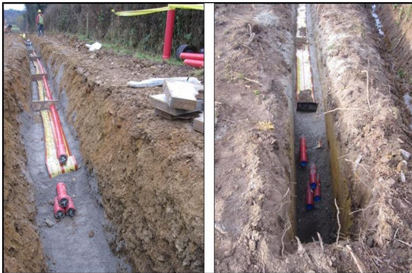
Figure 2.12 Typical Cable Trench (Extracted from CEMP)
